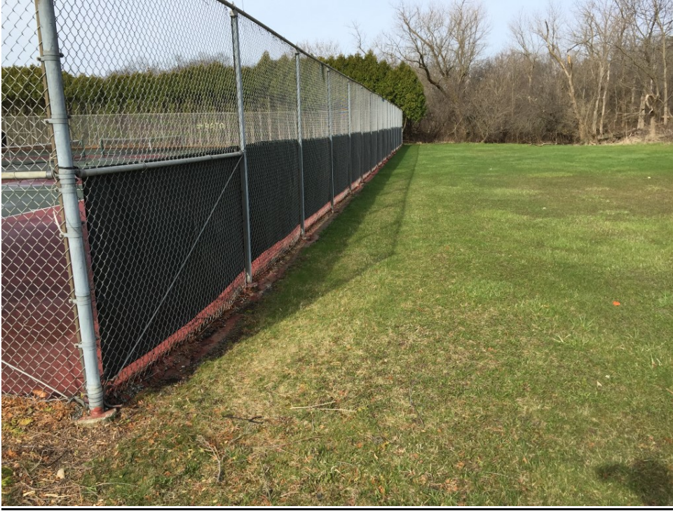
Photo 3 - Northeast Corner Looking West
