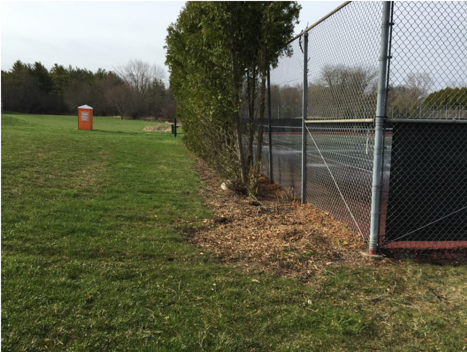
Photo 1 - Northeast Corner Looking South
