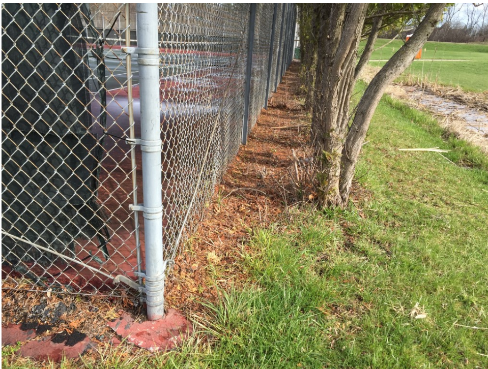
Photo 8 - Southeast Corner Looking North
